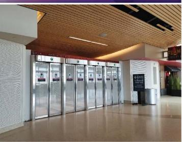
The Airport installed four high-tech one-way exit lanes at the south end of the Terminal B concourse, which enhances the flow of exiting travelers while maintaining the safety and security of passengers waiting for their flights. The exit lanes automatically open for people exiting but will sound an alarm if someone approaches from the opposite direction. If alarms are activated, the series of exit doors will not open until cleared by Airport law enforcement officers.
